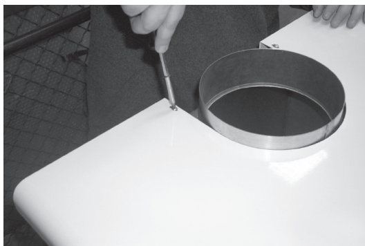
Fig. 6 - Unscrew the 2 self-tapped screws holding the boiler cover.
